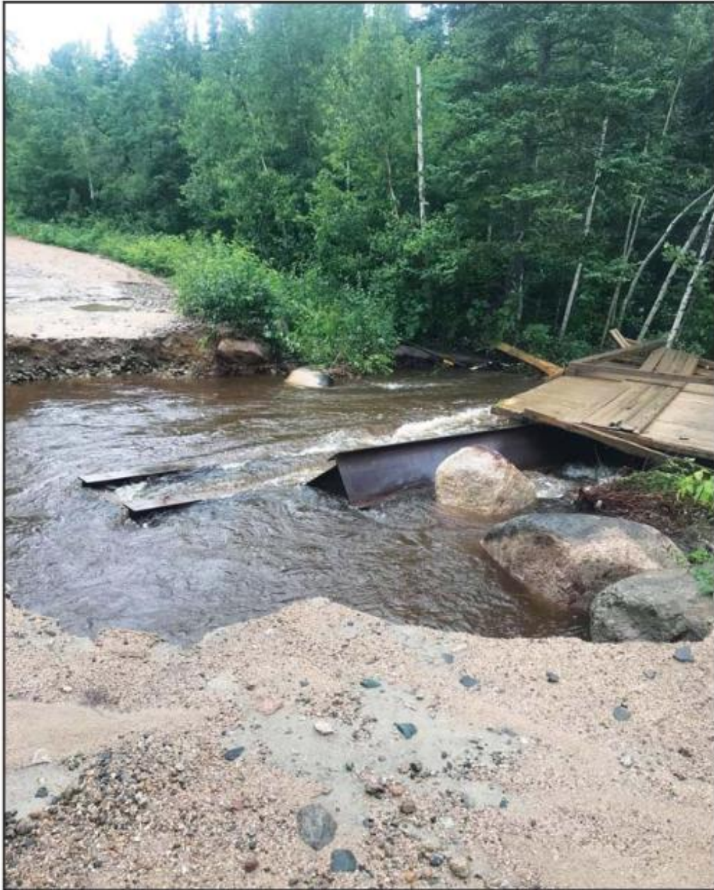
The southern section of the OHRV trail system in Jericho Mountain State Park was damaged in Tuesday's heavy rain. N.H. Trails Bureau officials were reported assessing the damage Wednesday. (PRESIDENTIAL OHRV CLUB PHOTO)
