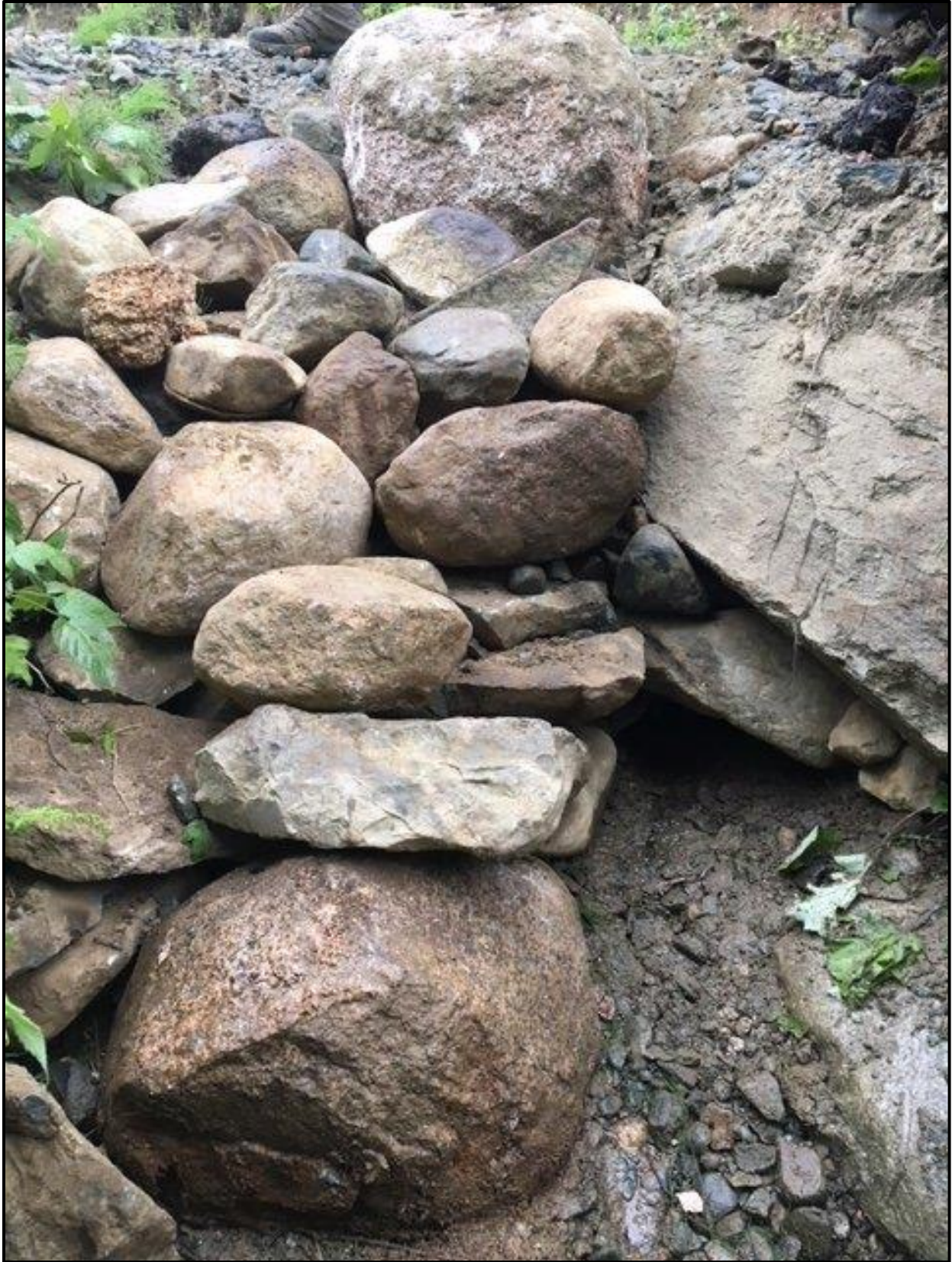
Finished rock stack.
