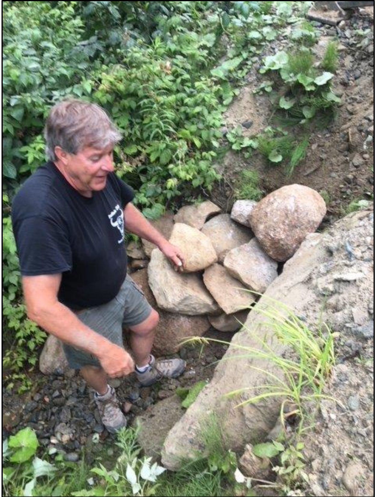
Steve stacks rocks into the washout by hand.
