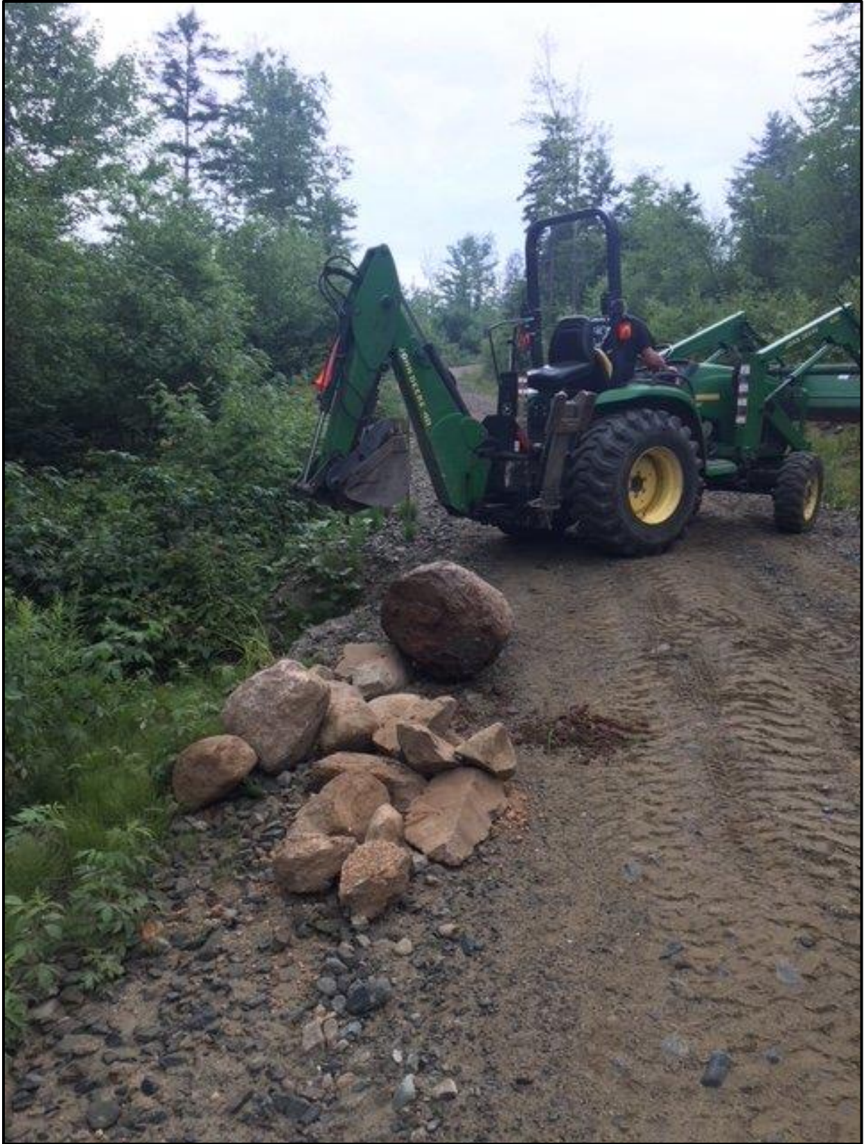
Steve uses his tractor to gather rocks to fill the washout.
